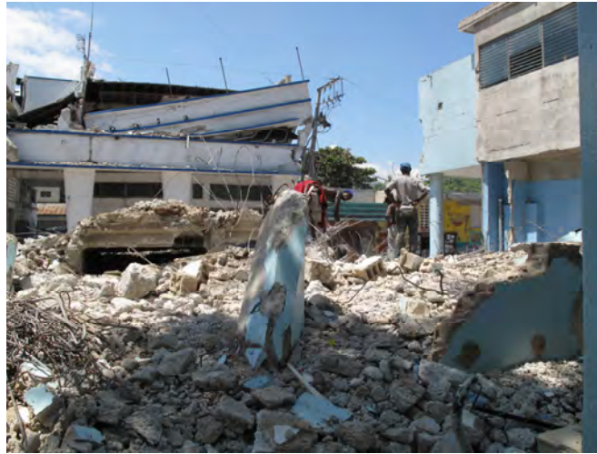
St Vincent Eye Hospital completely destroyed by earthquake
