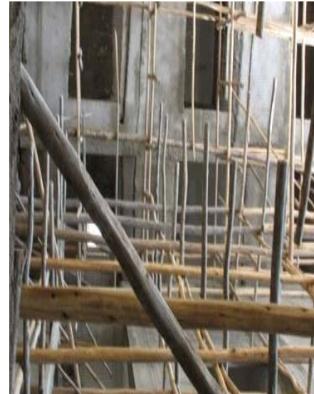
Scaffolding at new cancer hospital.
