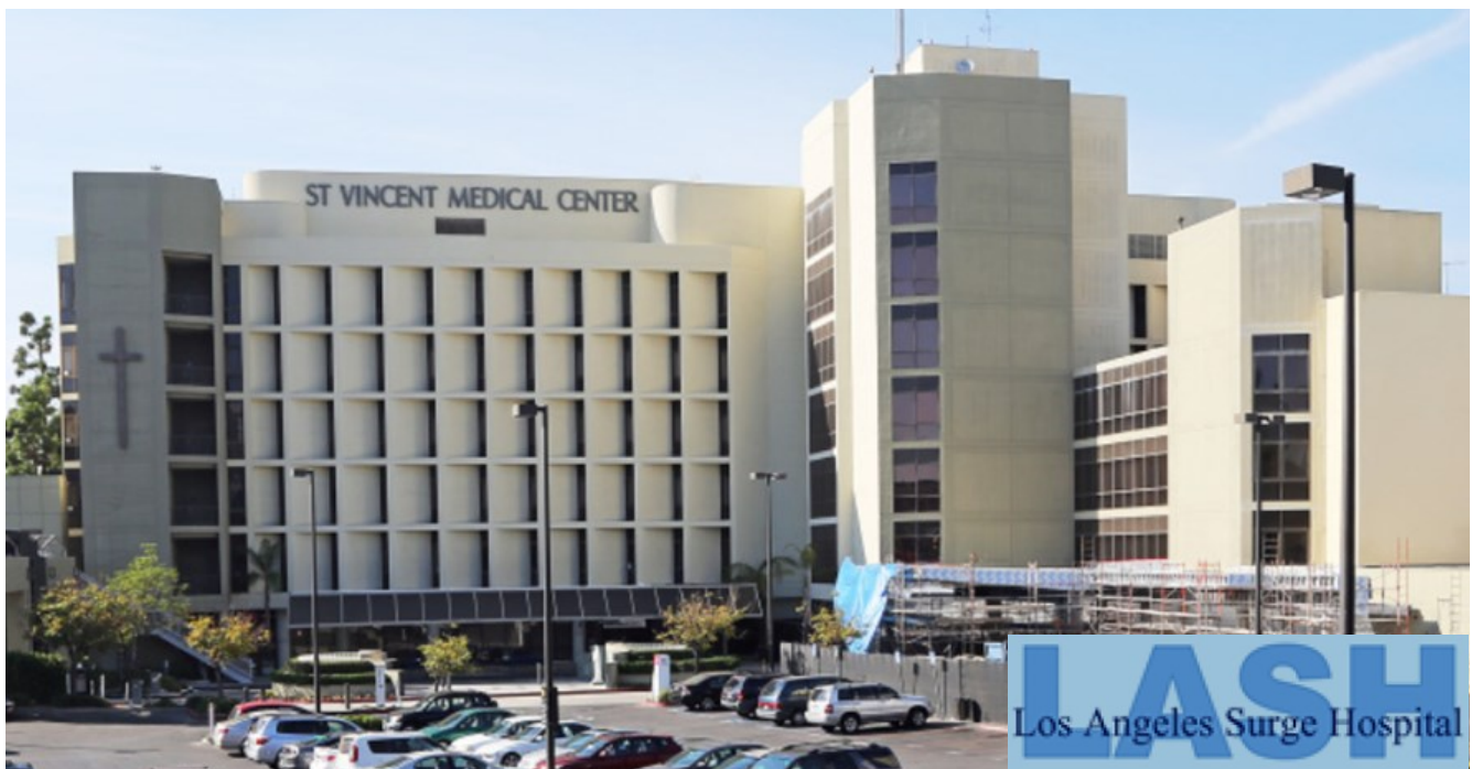
The previously closed and former St Vincent Medical Center in Los Angeles is being re-purposed as Los Angeles Surge Hospital by Kaiser And Dignity Health.
