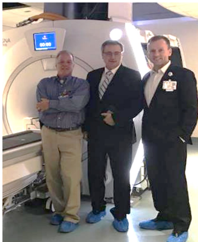
Donald Dunn, Stanford Childrens CE, George and Ilir at an MRI scanner installation
